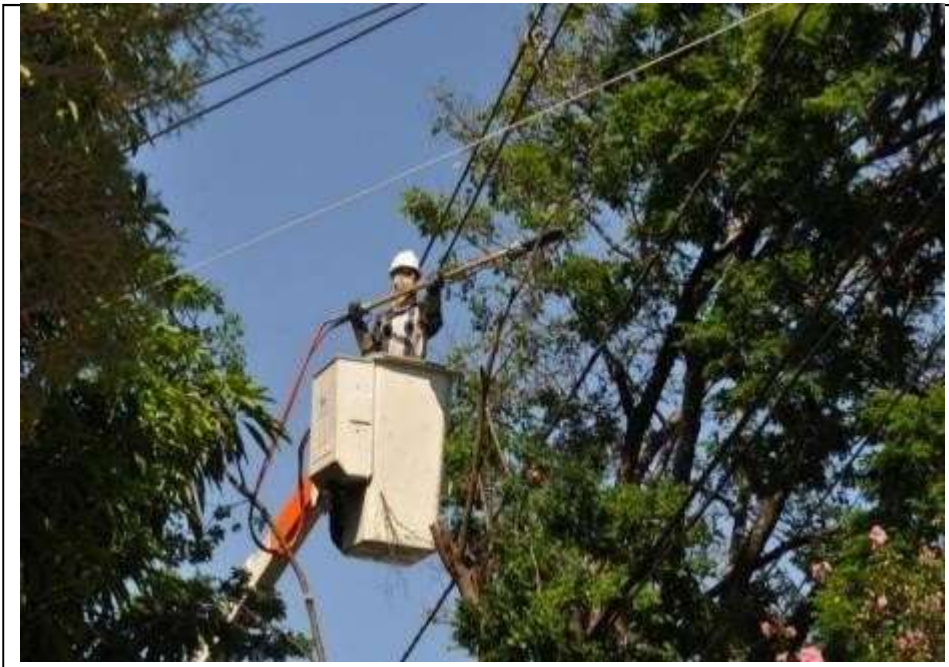
Figure 4: ELV executor in the activity of vegetation pruning.
